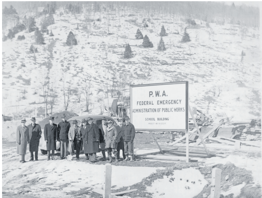
Photo contributed by DCHA, Fenton Collection. Building site of Margaretville Central School, 1939.
